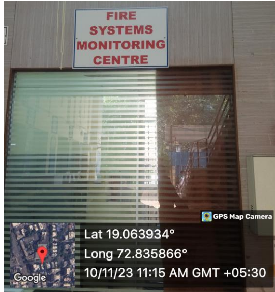
Fire Systems Monitoring Center (NB Ground Floor)
